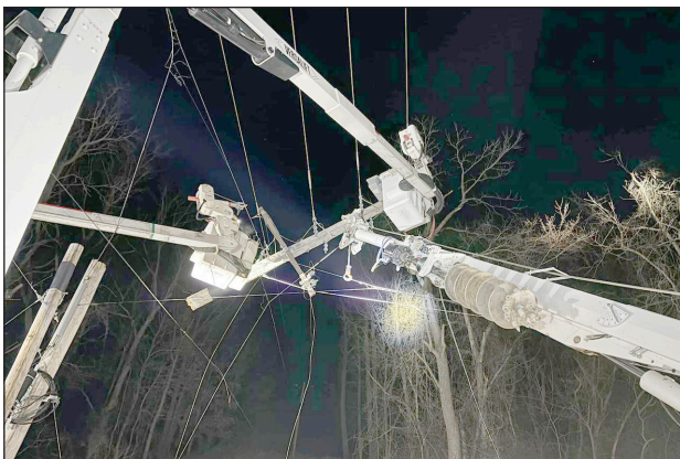
Barry Electric Cooperative lineman work to repair a broken three way pole on Saturday night near Oak Hill Cemetery. Photo: Barry Electric Coop
